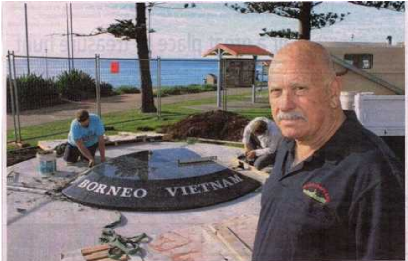
Small Ships veteran Bob Modystack oversees construction of the Small Ships memorial at Point Danger.
